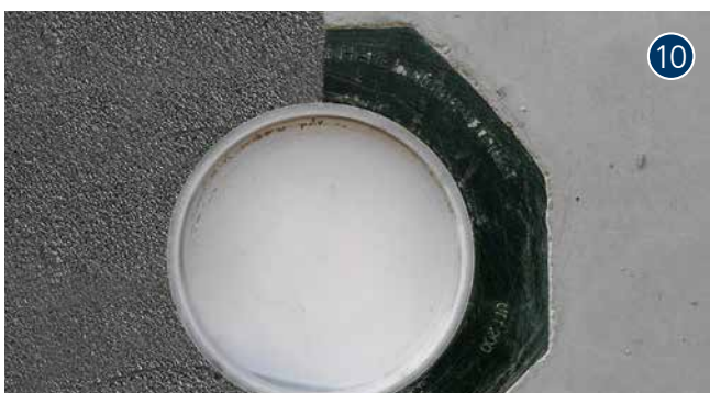
UFR concreted in a wall with PMBC
