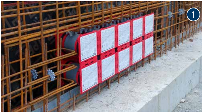
double wall insert HSI150 K2 before concreting
