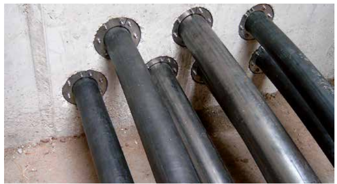
HRD press seals installed
