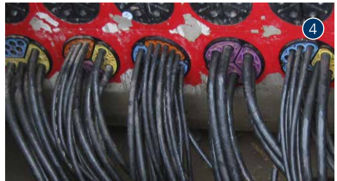
wall insert HSI150 S3 with SEG segments
