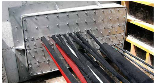
rectangular split flange for several cable penetrations
