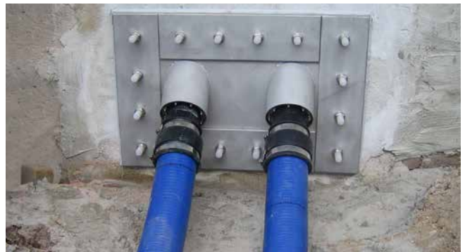
fixed/loose flange with slanted empty hose connection and surface sealing
