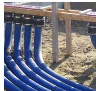
side by side arrangement 2x KES150 MA ZVR150/500 on the installation fixture KES FUBO-FIX AV
