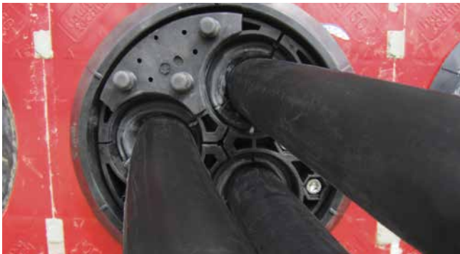
pressure plate cover HSI150 DG PA 3x24-54
