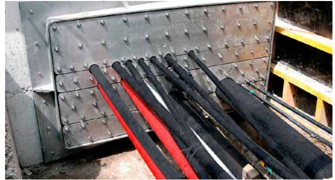
split rectangular flange with multiple cables
