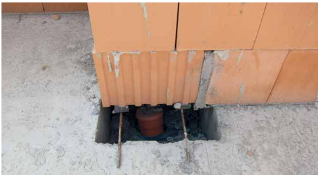
difficulty: retrofit gas-tight and vapour-proof sealing
