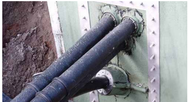
split fixed/loose flange according to DIN 18533
