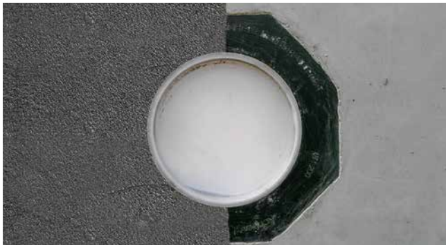
concreted UFR with PMBC
