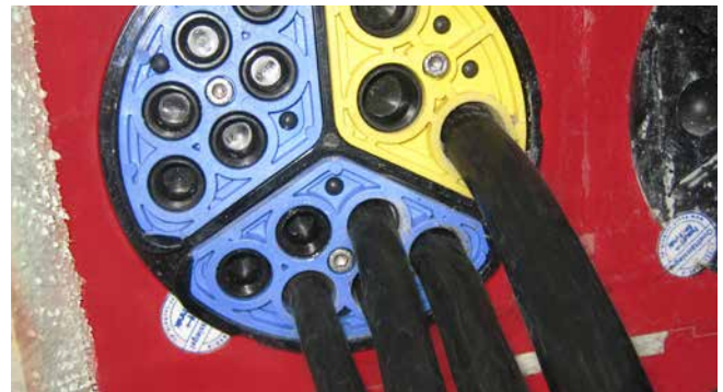
HSI150 SEGMENTO with integrated torque control system and blind plug
