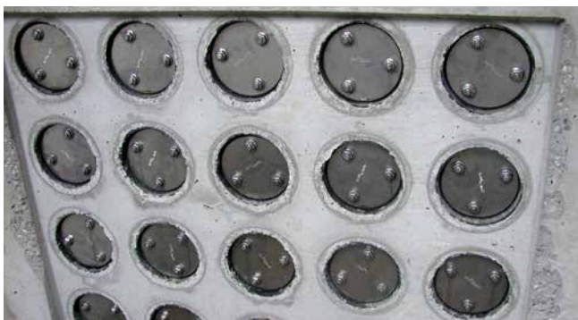
FZR100/240 – pipe section sealing
