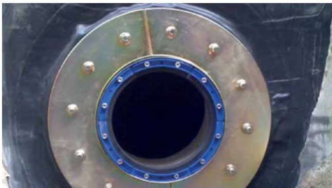
FLFE 1x300/X A3C with the standard press seal HSDC (powder-coated)
