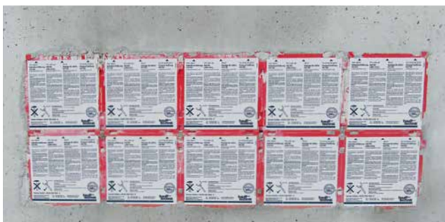
double wall insert HSI150 as block assembly
