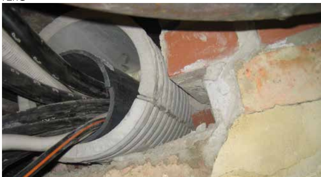
FZRG150/350 – refurbishment in masonry
