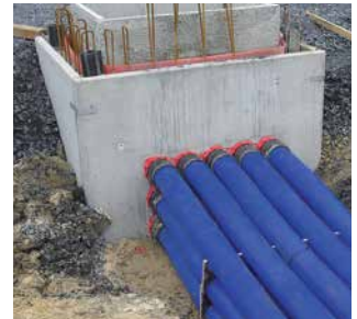
KES MA90 D – connection to the HSI90 wall insert
