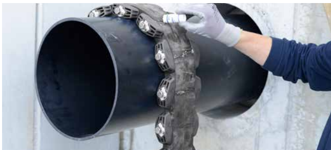
GKD400 – installation preparation with lubricant GM
