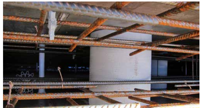
ZVR200/300 fixed in formwork
