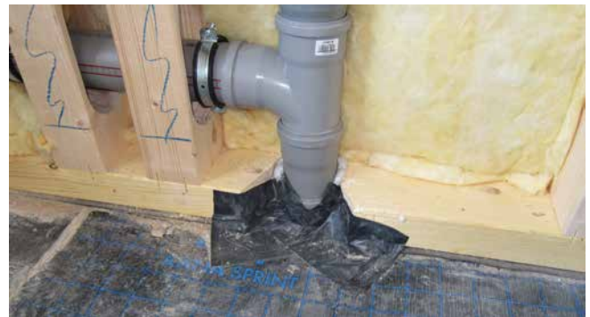
difficulty: integration of vapour barrier foil
