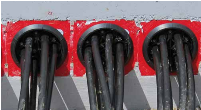
low-voltage cables sealed with HSI150 DG 6x10-36
