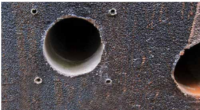
core drill and dowel holes
