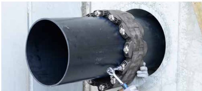
GKD400 – tightening of segments
