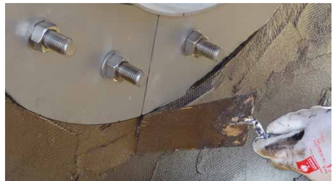
FLFE 1x300/X stainless steel design with connection to PMBC by means of fleece inlay
