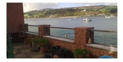
Visual impacts of tidal and river defence walls are a sensitive issue, as they partially block the impressive sea or river views. Incorporating flood defence glazing resolves objections to schemes raised by local residents, whilst still achieving the required wall height and protection. Flood defence glass walls prove a popular solution with the local communities, helping to minimise the visual impact of schemes.
