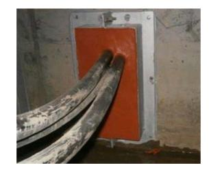
The existing cable entries and ducts around and beneath a building present a clear risk of water ingress during a flood. This is a particular issue for buildings housing large and high voltage electrical equipment, such as a substation switch room, which often will have tens if not hundreds of cables fed through below ground level and terminating inside the building.
