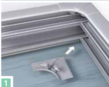
1 Install the upper and lower parts of the angles on the trunking
