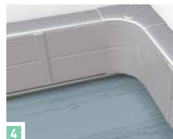
4 Finish the installation by clipping the rigid covers across the whole length of the trunkings
